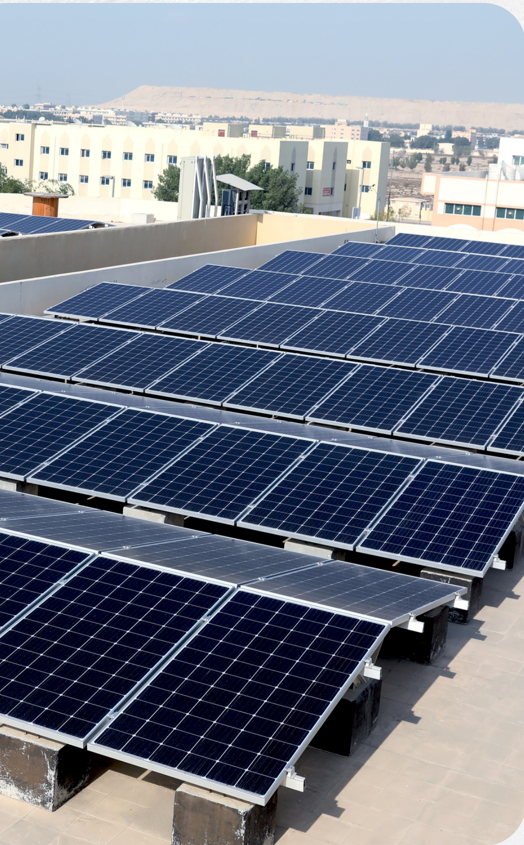
Solar panels on the rooftop of one of Transguard Group's accommodations
